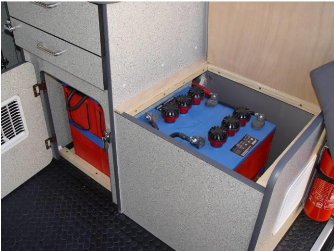
Power supply by battery pack
